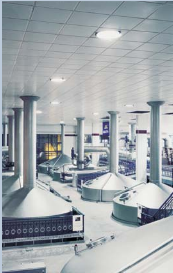
Huppmann plant engineering as far as the eye can see – in the Baltika brewhouse in St. Petersburg
