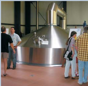
On the Open Day at the Kulmbacher Brewery festival the public could learn about the wort boiling system.
