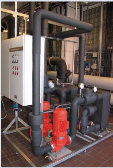
Efficient CO 2 recovery.
