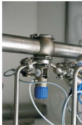
In the system at Weißbierbrauerei Schneider, cleaning and sterilisation is integrated in the piping and the process flow.
