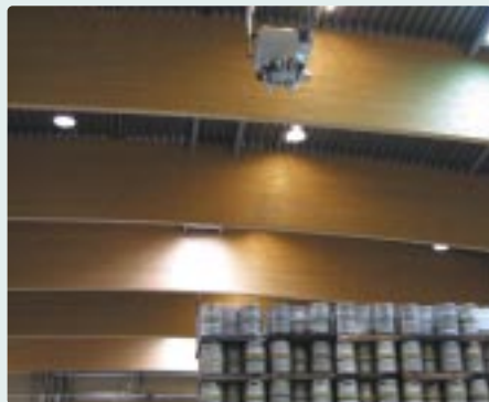
Inside the warehouse showing the headroom, as yet unused auxiliary heating and the huge 2-metre high Glulam support beams.
