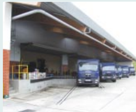
The loading bay for the local delivery fleet. Note the large bore pipes to collect rain water from the roof.
