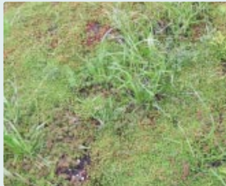
Detail of the low growing sedum roof covering.
