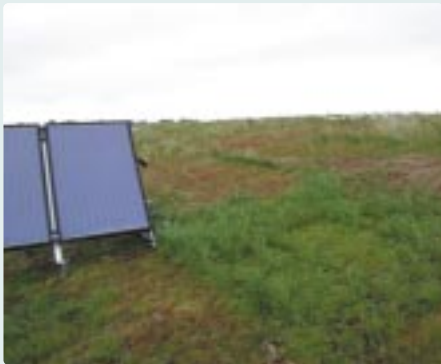
The gently arched roof showing the sedum and some ferrule grasses as well as a small set of solar panels to heat the hot water.
