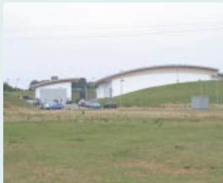
A long shot with cellar services and vehicle workshops on the left and the huge span of the main warehouse on the right.
