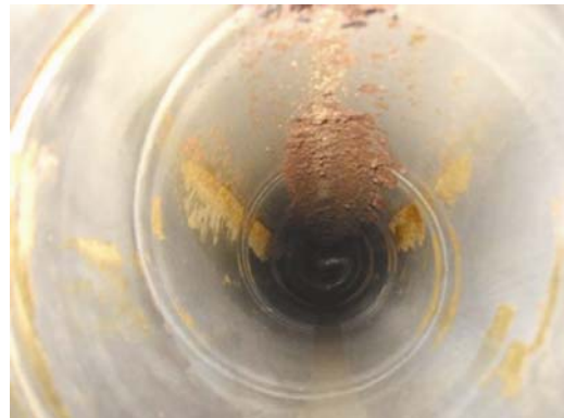
Figure 6. Inner pipe surface after cleaning.
