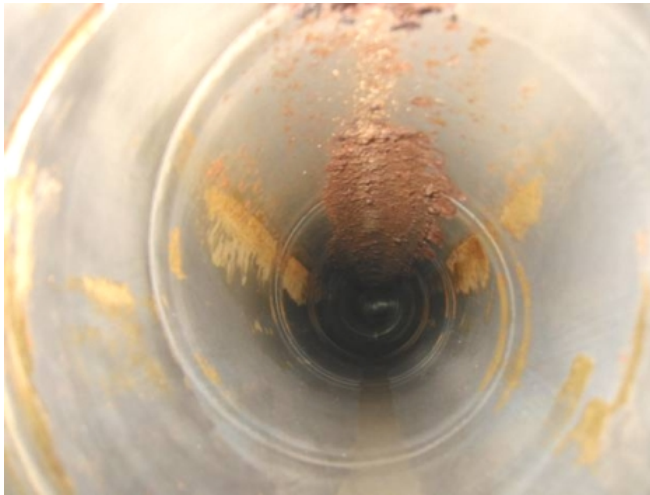
Figure 5: inner surface of the pipe after cleaning
