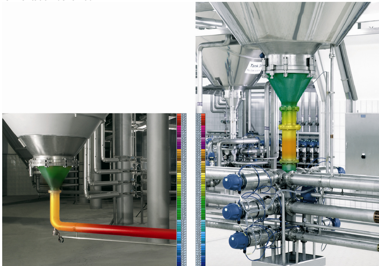
Figure 1: temperature distribution in the pipe in comparison (left: conventional tank outlet, right: ECO-MATRIX)
