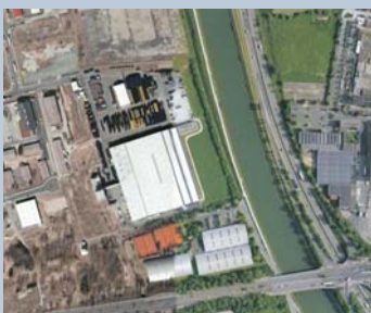
From the air, the new brewery can be easily recognized by the already existing logistics centre (white). The Main-Danube Canal runs directly next to the brewery (Picture: Google Earth).
