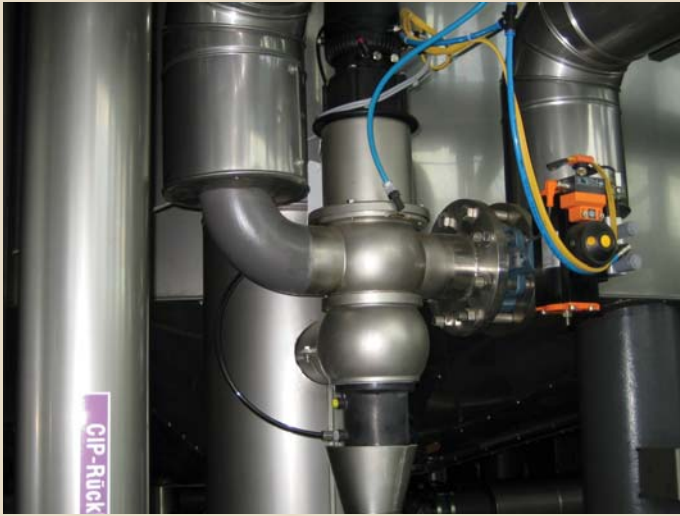
Fig. 4 A double-seated valve is used to direct flow during wort precooling
