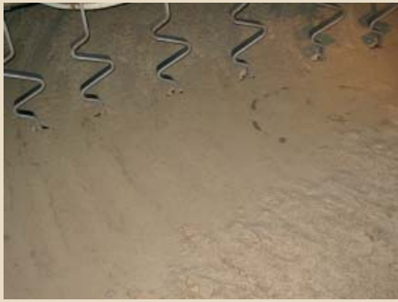
Fig. 1a Uneven spent grains bed with the old side inlet
